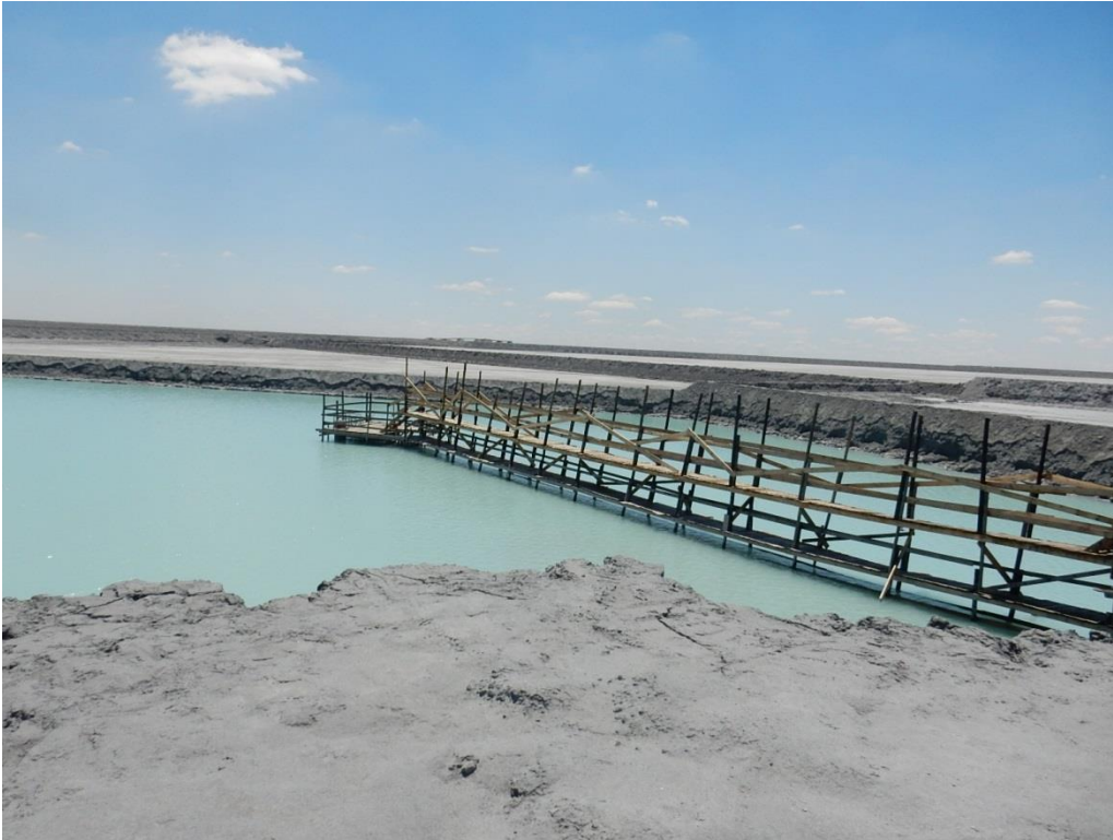
Access walkway at penstock inlet tower on ash dam 5
